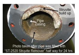
As digestors and waste water plants handle millions of litres of water these products combine and form Struvite under the right conditions.
